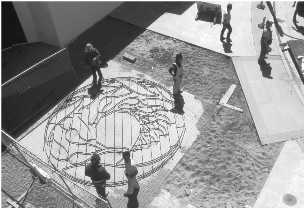
ABOVE Construction workers frame in the Aquarium's kelp logo that still greets visitors outside our main entrance.
